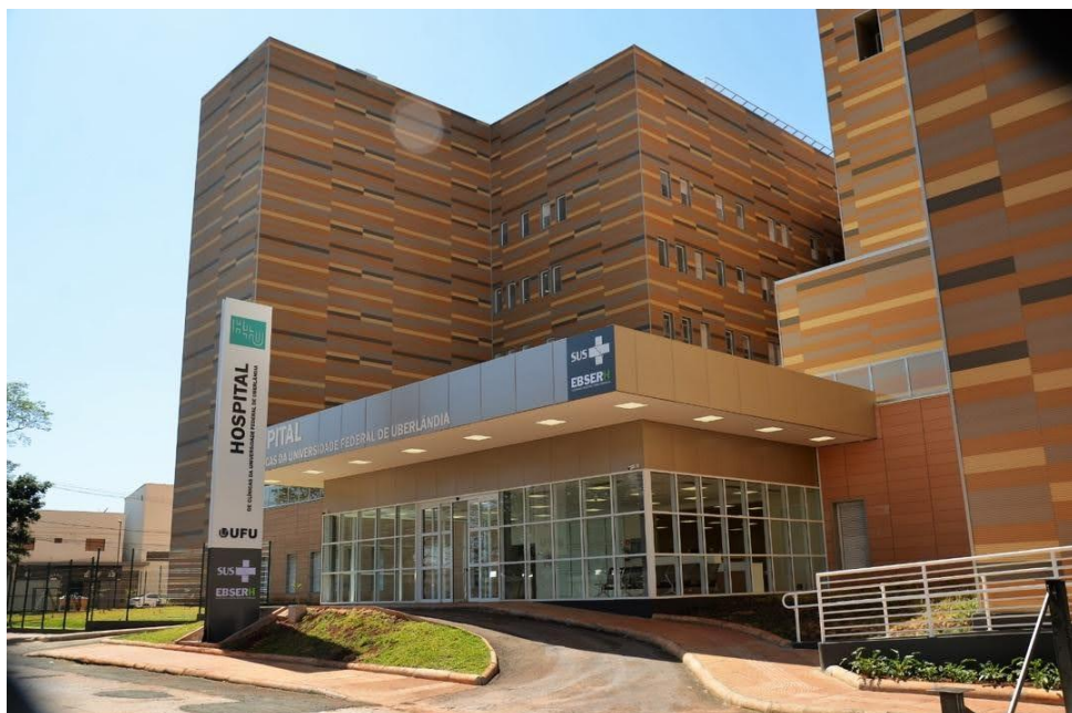
Figura 17-Entrada principal hospital novo
